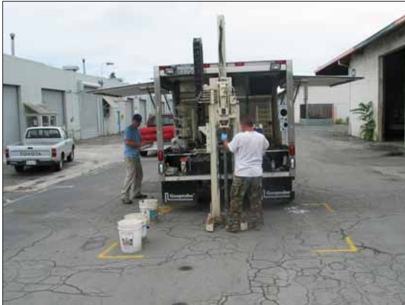
Figure 18. Coring to explore subsurface deposits.
