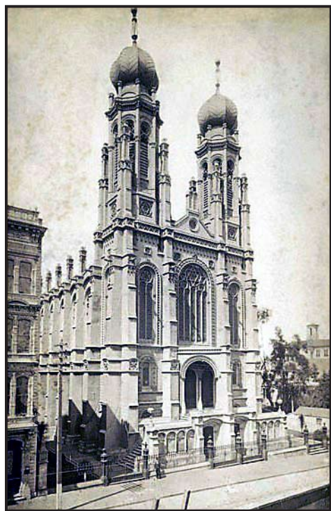
Figure 8.4. The Sutter Street Synagogue. This 1866 building was home to Congregation Emanu-El. The building is an interesting marriage of church-like architecture and subtle Jewish symbols. The Magan Dovid (Star of David) is displayed significantly above the line of sight, while the twin domes evoke the crowns ( keterim ) used to decorate the etz chaim , the wooden handles of the Torah scroll. (Photo courtesy of the California History Room, California State Library, Sacramento, California)
