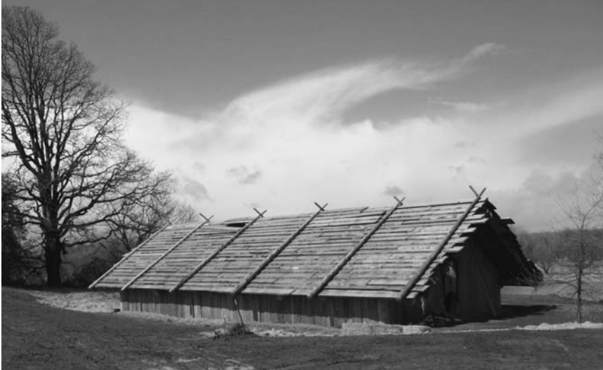
Figure 2 Chinookan plankhouse constructed on the grounds of the Ridgefield National Wildlife Refuge
